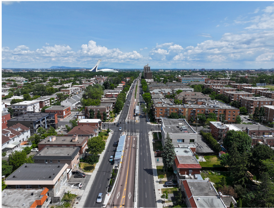
Fig. 3. Picture of the Pie-IX BRT infrastructure (Source: Authors).
